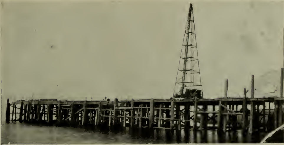
FIG. 6A. WOULDHAM CEMENT CO.'S UNLOADING JETTY.
